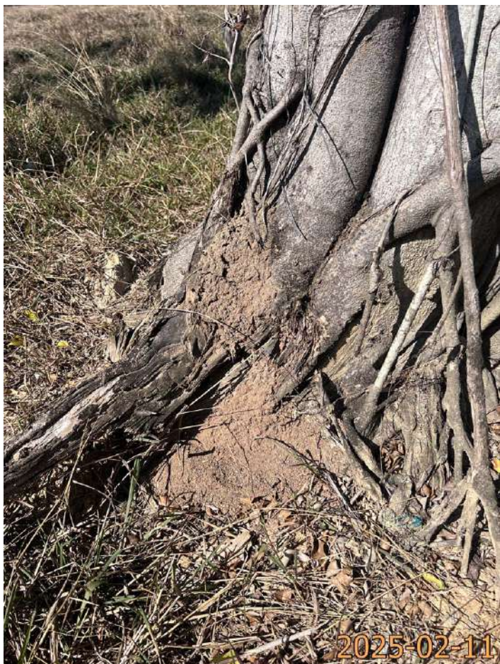
T17 Trace of termite
